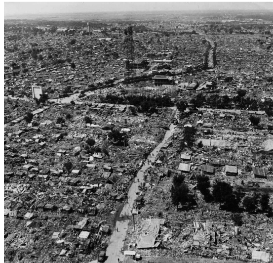
Figure 12 Photo showing nearly complete devastation in the Lunan district of the city of Tangshan from the 1976 Tangshan, China, earthquake b0360 (Huixian et al. , 2002). Tangshan was a major industrial center with a population of 1 million before the earthquake, which occurred directly under the city at 3.42 a.m. About 93% of residential buildings and 78% of commercial buildings in the city were destroyed b0965 (Yong et al. , 1988). The officially reported death toll is 255 000, but estimates are as high as 655 000. f0060
