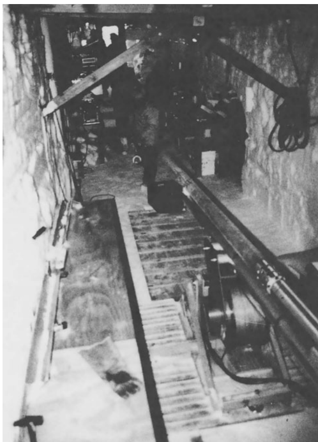
Figure 8. Ice-core activities on James Ross Island ice cap, Antarctic Peninsula. The drilling operations were developed in a large trench dug in the snow, used as protection from the extreme climatic conditions.
