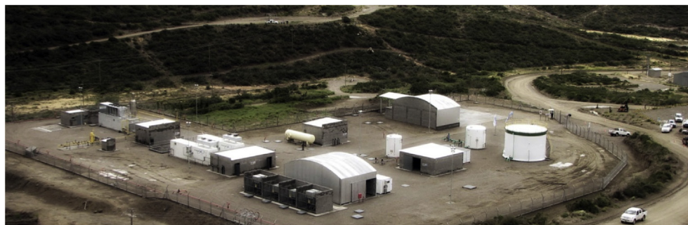
Fig. 9 – Hychico wind park & hydrogen plant.
