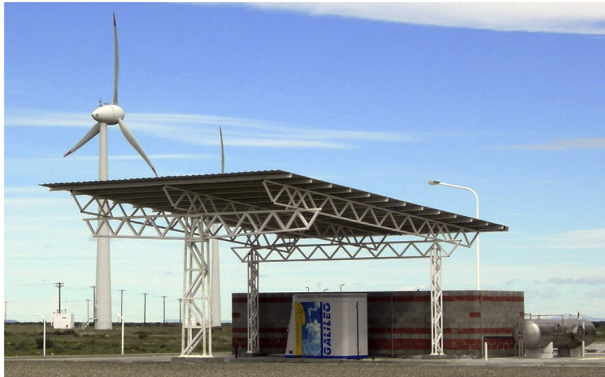
Fig. 7 – Fuelling station at the Pico Truncado plant.
