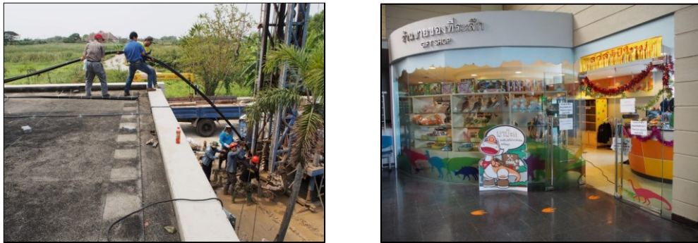
Figure 3. Installation of ground heat exchangers in Geological Museum, Department of Mineral Resources of Thailand
