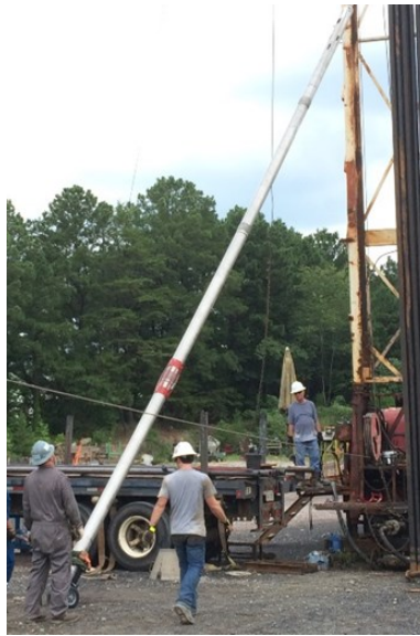
Figure 1 Olympic Research ceramic plug tool emplacement field test.
