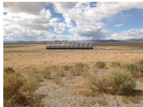
(b) Geothermal power plant (AltaRock, 2013)
