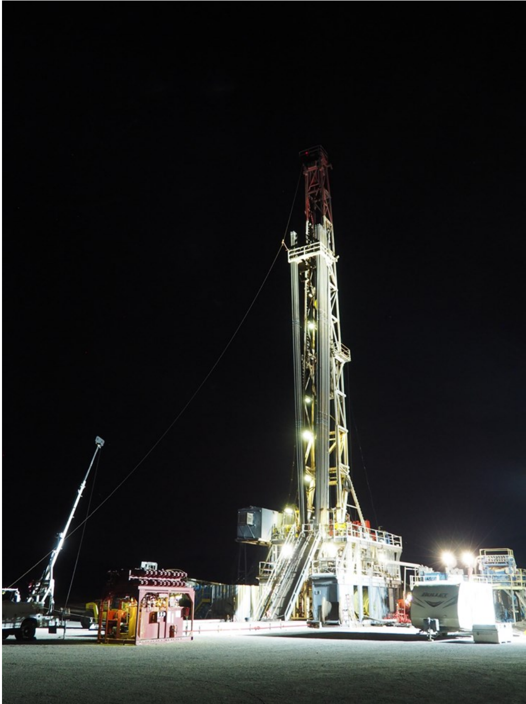
Figure 4: View of the drill rig, with boom of the temperature logging truck on left.
