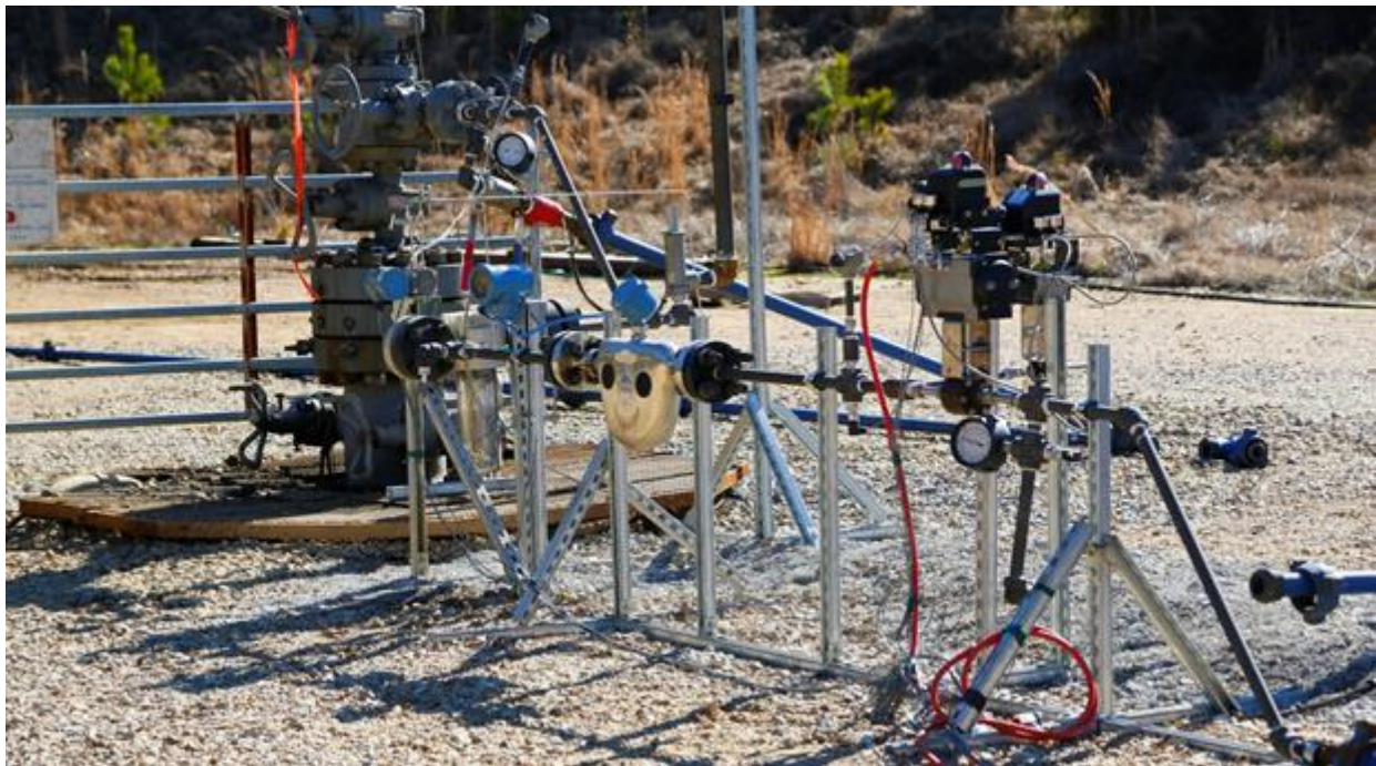
Figure 8. F3 production well with computer actuated valve system and Emerson Micromotion Coriolis mass flowmeter to control and monitor the CO 2 production. F3 wellhead can be seen in the background.
