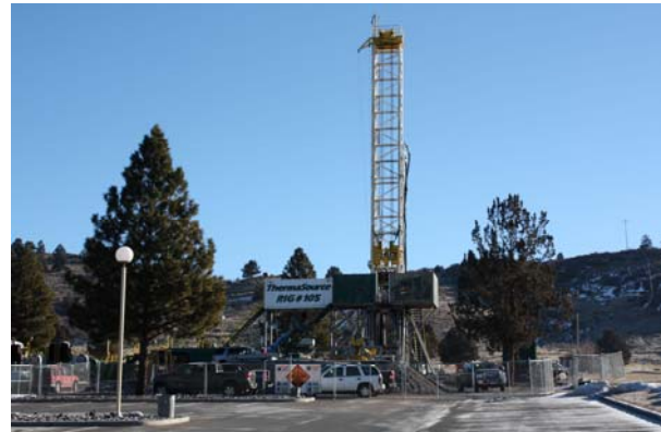
Figure 8: ThermaSource drilling rig on the OIT campus.
