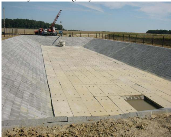
Figure 4: Construction of a 2000-cubic-meter pit.
