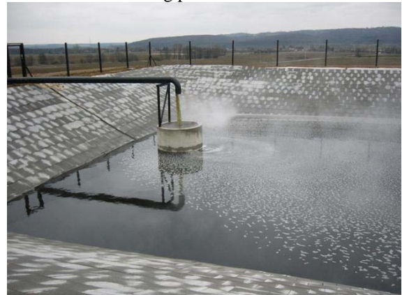
Figure 5: Thermal water test production from a layer of 142°C temperature in Hungary
