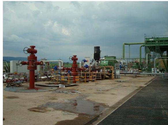
Figure 8. The 3 well-heads on the geothermal platform with GPK4 (left), GPK3 (middle) and GPK2 with the external black motor of the LSP (right).
