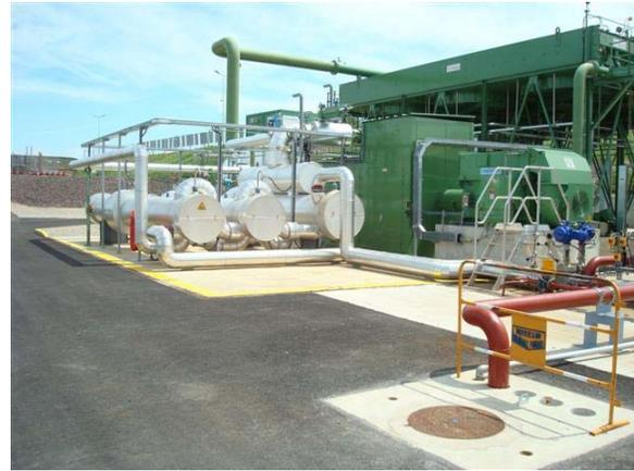
Figure 10. The ORC part of the Soultz power plant. On left, the heat exchanger. On right the generator and the air cooling system.
