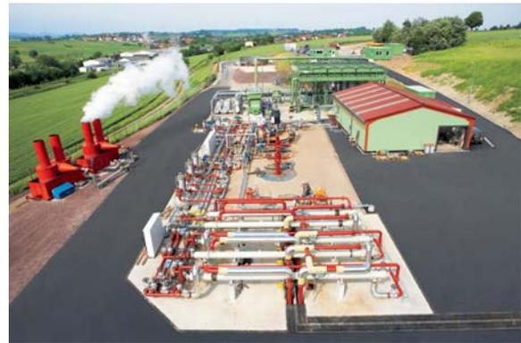
Figure 11. The Soultz geothermal power plant: in the back, the ORC power unit; in the middle, the 3 geothermal wells; in the front, the cooled geothermal loop.
