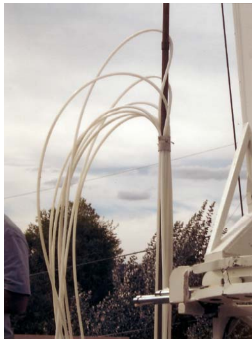
Figure 7: Placing the promoter pipe and PEX tubing into the well.
