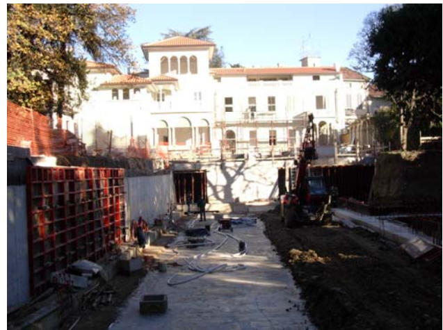
Figure. 2. Boreholes field for a IXX cent. Villa restoration
