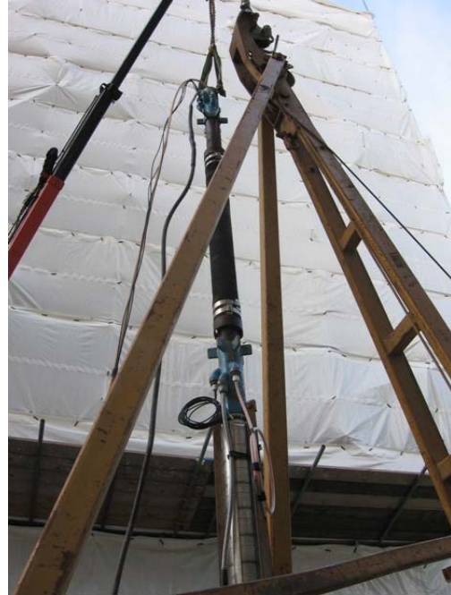
Figure 4. Equipment being lowered into the borehole
