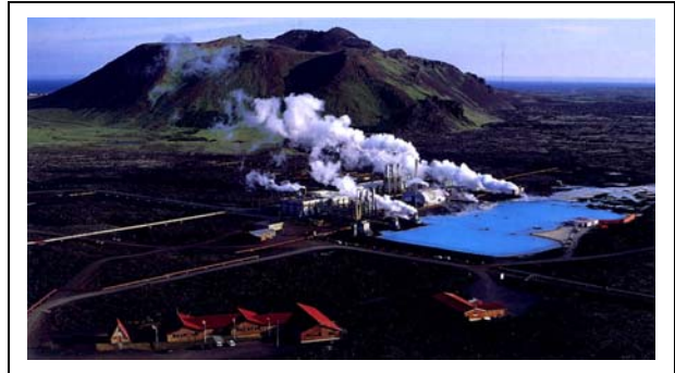
Figure 16. Combined heat and power plant at Svartsengi, Iceland – Blue Lagoon on right (courtesy of Haukur Snorrason, Rekkjavik, Iceland).
