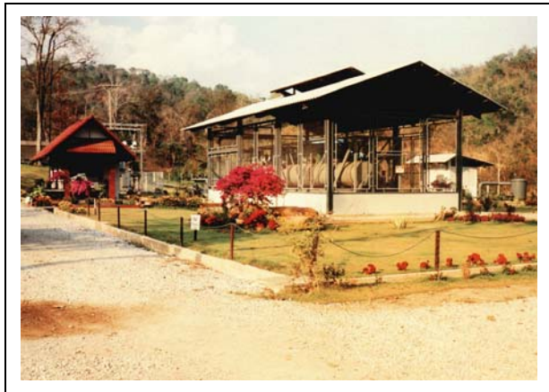
Figure 18. Binary power plant, 300 kW, at Fang, Thailand.
