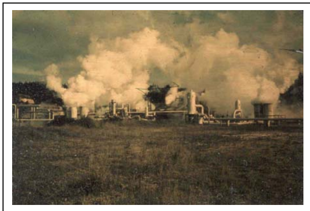
Figure 9. Wairakei, New Zealand geothermal field.
