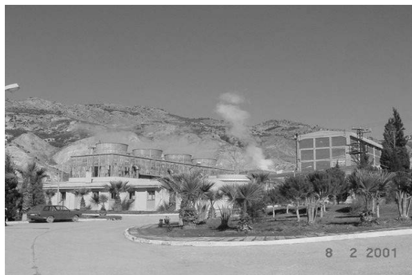
Figure 2: Kizildere geothermal power plant
