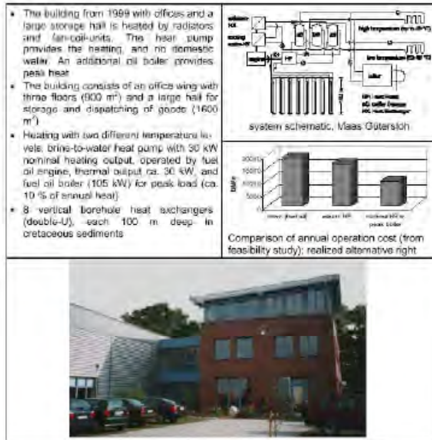
Fig. 9: Commercial building “Maas Naturwaren” in Gütersloh
