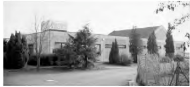
Fig. 1: “Verolum”-building in Schwalbach south of Wetzlar, first GSHP with BHE in a commercial application in Germany, built 1980, photo from 1995; the BHE are located beneath the bushes to the left and front of the building
