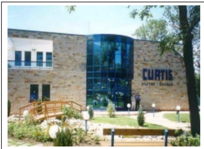
Figure 3. Space heating, air-conditioning and ventilation (Curtis-Balkan Ltd, Sofia City)
