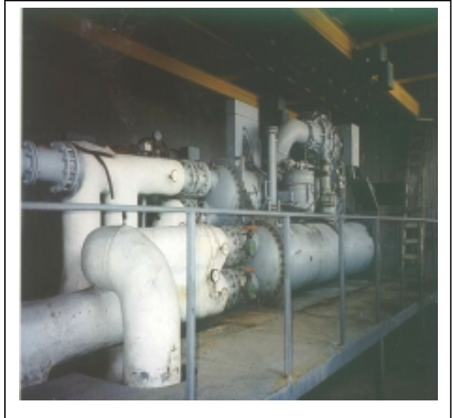
Figure 2. Heat pumps installation in "Golden sands" resort, (Northern Black Sea coast)
