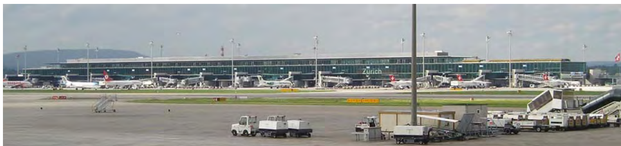
Figure 1: The Dock Midfield of the Zürich airport has been built on 440 foundation piles of 30m.
