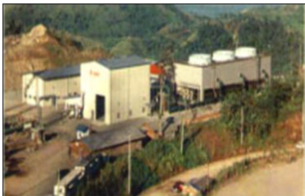
Figure 11: Leyte Binary Plant.
