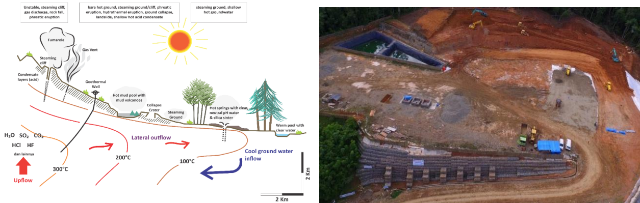
Figure 7: Left: Simplified diagram of the geothermal system in high-relief terrain such as Indonesia (Utami, 2010). Right: Installation of gabion wall in a well pad to anticipate the landslide caused by the slope.
