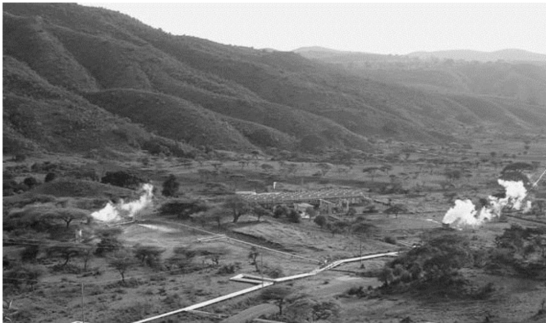
Figure 3: Aluto Langano Gpp in Operation
