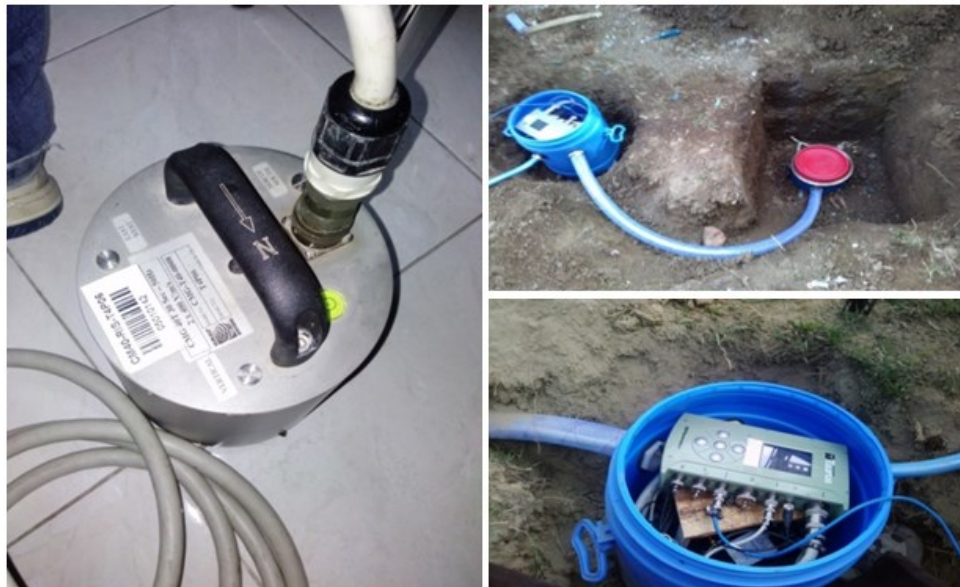
Figure 2: A figure showing Seismometer installation processes.
