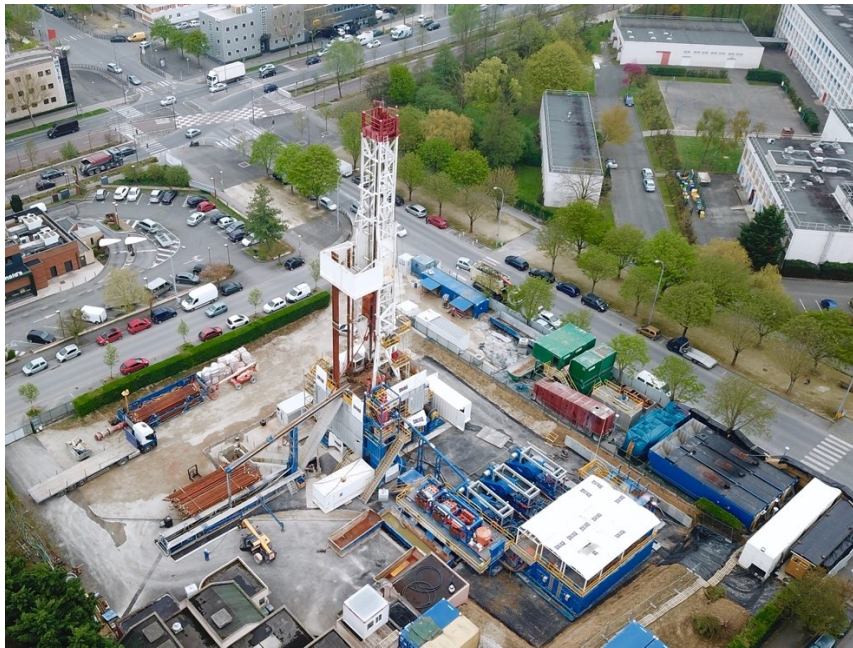
Figure 6: Geothermal well drilling at Bonneuil-sur-Marne, Paris, France (source GPC IP)
