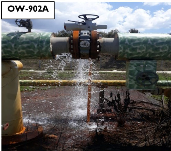
Pictures showing the effects of low condensate pH on the condensate re-injection wells.
