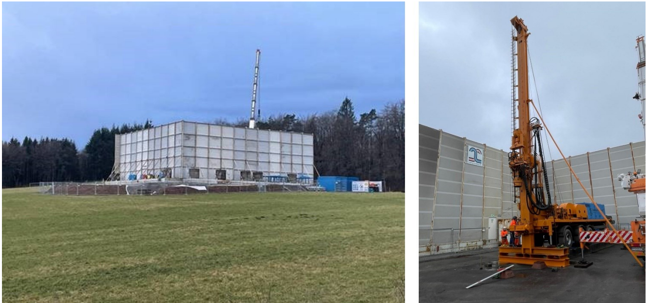
Figure 2: Preparation of the drill site for the first exploration well GLB-1 with the drilling site being protected with a noise barrier and the drilling rig.
