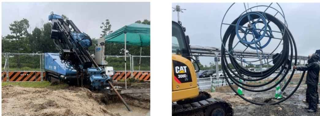
Figure 1: HDD equipment used for the horizontal GHE in Saga City
