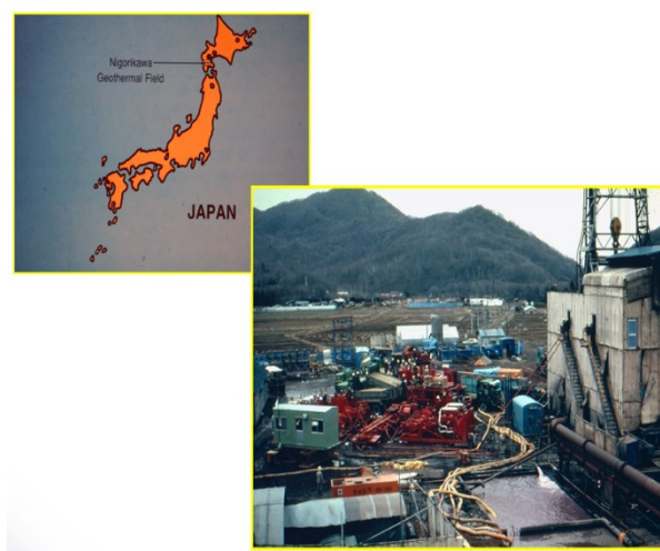
Figure 8: Frac spread at a Nigorikawa Geothermal Field well
