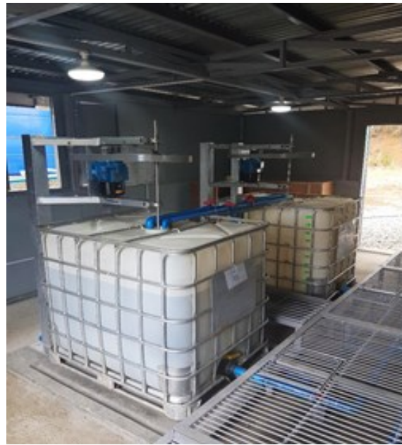
Figure 4: Fabricated mixing tanks used to attain a homogenous solution of desired concentrations of NaOH.
