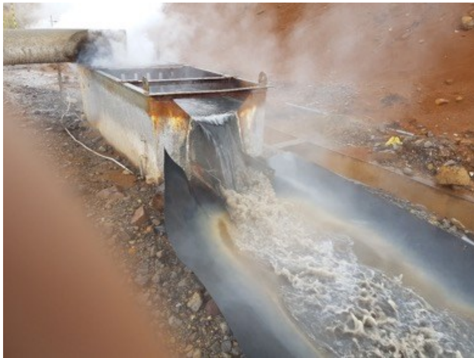
Figure 14: Dark discharge out of the weir box of BN-06D near the end of the FMS test.
