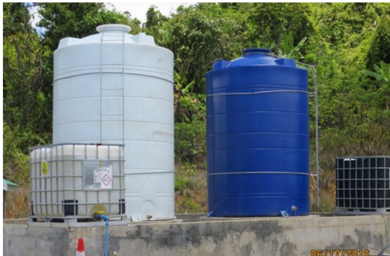
Figure 3: Storage tanks used for caustic soda (white) and water (blue). Both are made up of polyethylene material with UV stabilizers.
