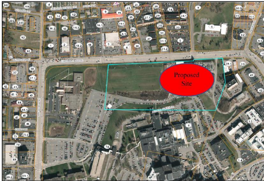
Figure 1: The aerial view of the proposed geothermal well site location on WVU Campus.
