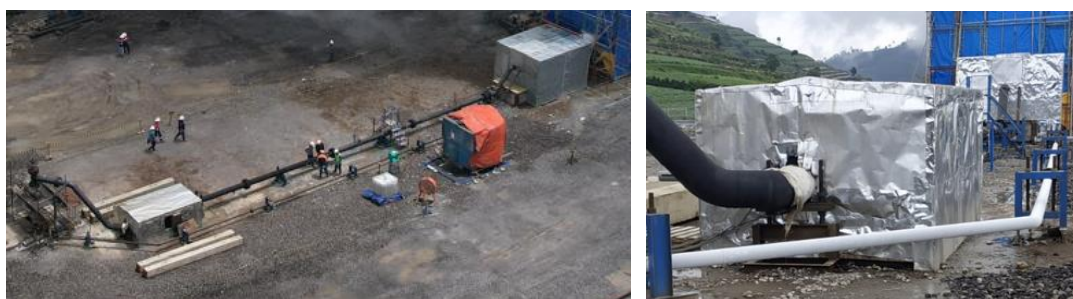
Figure 6: Sound Barrier Implementation in Dieng
