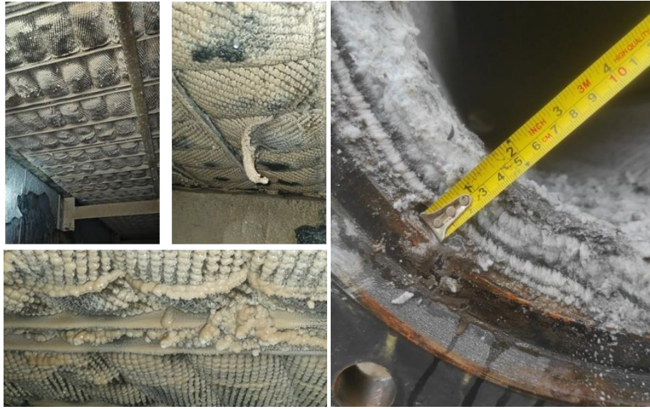
Figure 9: Mist Pad Condition after plugged by Silica (left); Silica deposition at brine manifold (right)
