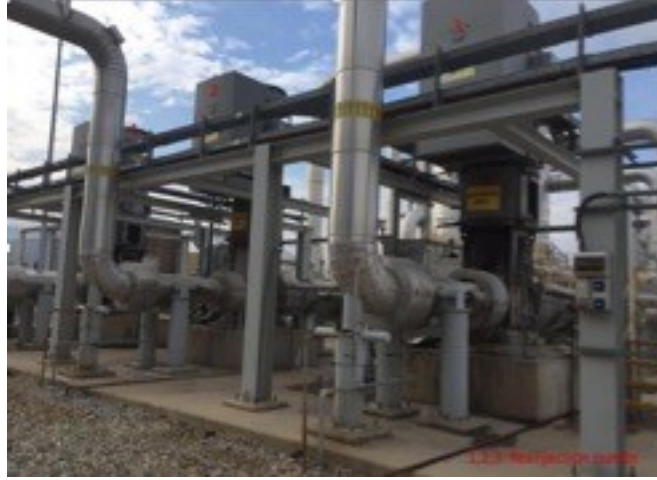
Figure 4: Re-injection pumps in Alaşehir-1 GPP (Photo credit: Zorlu Energy Company)
