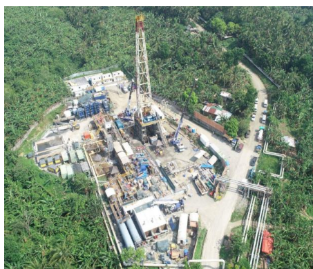
Figure 11: Simultaneous drilling and construction of surface facilities (piping works) at Well Pad P A
