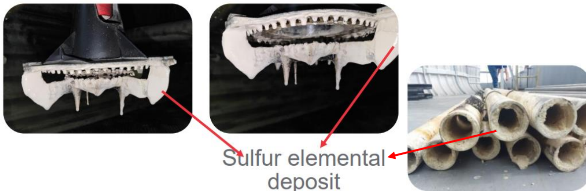
Figure 8: Sulfur deposit in the main cooling water system, mainly in cooling tower equipments
