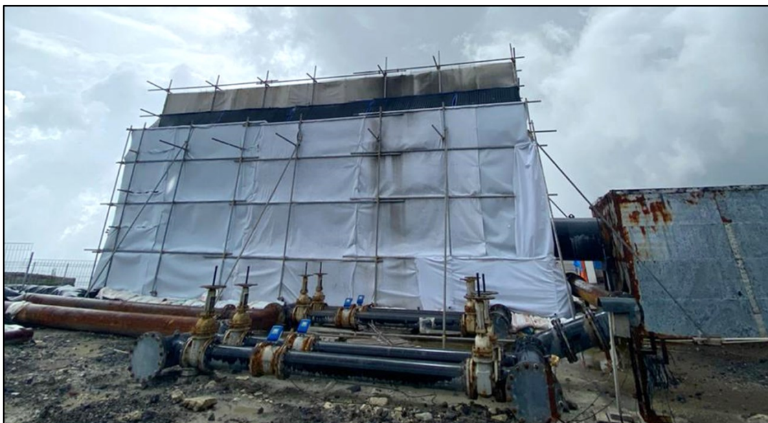
Figure 9: Sound barrier is installed to reduce the noise level around the well pad during well discharge test
