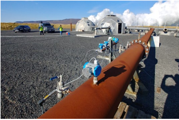
Fig 5. Orifice Meter Downstream of Well Head.
