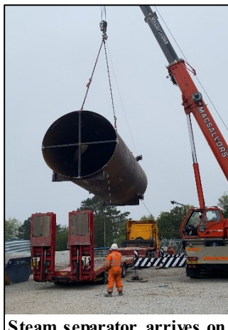
Steam separator arrives on site for installation
