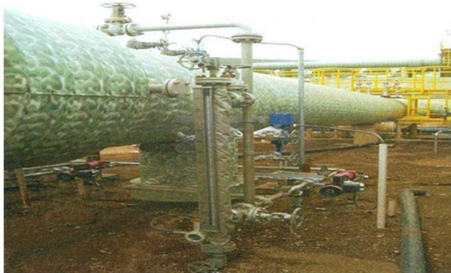
Figure 5: One of the CDPs with a level control system in Olkaria IAU
