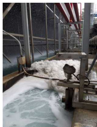
Figure (e) Foam Condition of CT Basin
