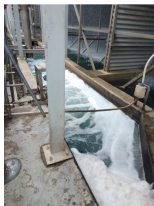
Figure (e) Foam Condition of CT Basin
