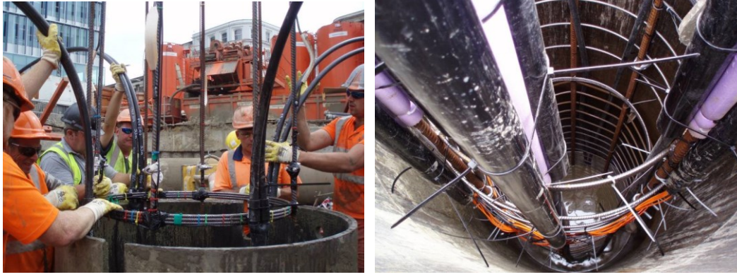
Figure 9: Installation of geothermal loop into the energy pile (courtesy of Kenichi Soga)
