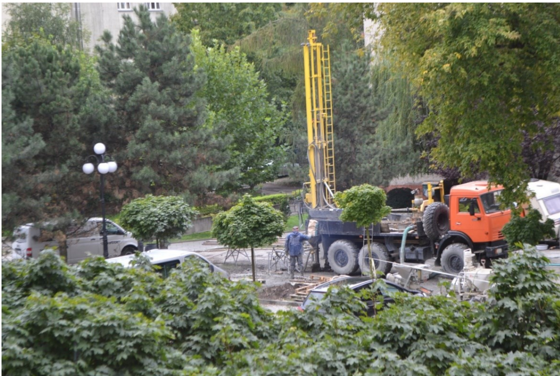
Figure 7: Drilling of new borehole heat exchangers at AGH UST in 2017 (Field B).
