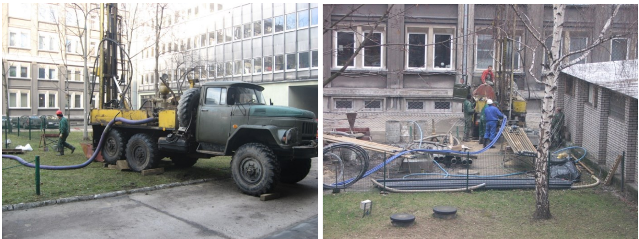
Figure 5: Creation of borehole heat exchangers on the AGH UST premises.
