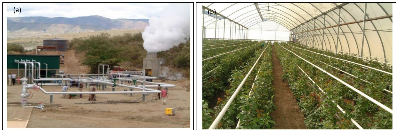
Figure 6: (a) Oserian heat exchanger system harnessing geothermal fluids from well OW-101. (b) Pipes running within the greenhouse to circulate hot fluids (Mburu, 2014).
