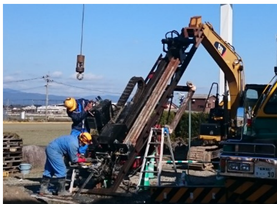
Figure 1: HDD equipment used for the horizontal GHE in Saga City
