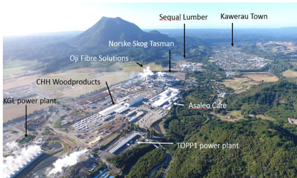
Figure 1: The Kawerau Industrial Complex in 2018 (three binary cycle power plants not in photo)
