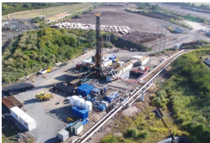
Figure 6: KA47 work-over using the Nova-1 rig.
