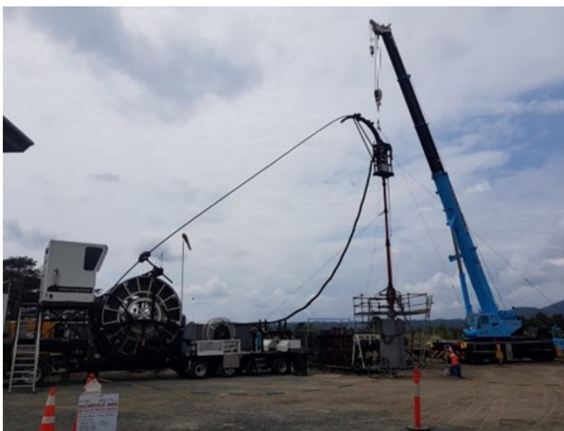
Figure 9: KA27 mechanical clean out using a coiled tubing unit.
