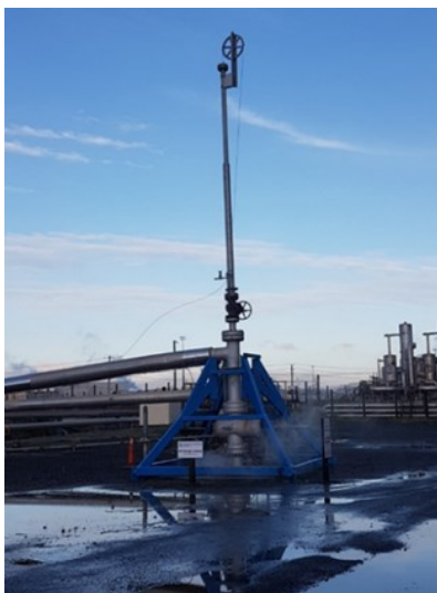
Figure 7: KA47 after well repair and anti-scalant system upgrade.
