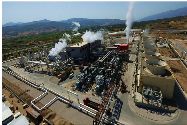
Photo.1 : Kizildere II triple-flash and binary system (Photo by Zorlu)
