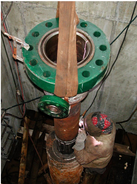
Figure 2: A new flange is welded on to the old casing.
