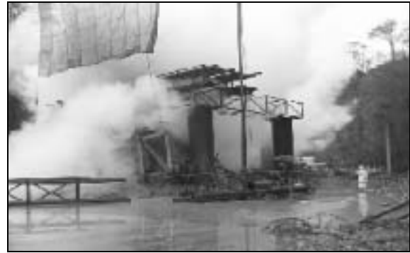
Figure 4. View of the Fabricated Discharge Diffusers and the Net (taken when Well 5R-12D was already partially quenched)
