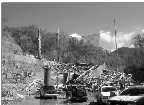
Figure 7. View of Well 5R-12D after it was totally contained.
