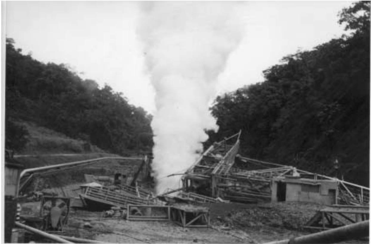
Figure 1. The uncontrolled discharge in well 5R12D that sent steam rising some 50 m above the well. On its side is the fallen rig and debris from the well.
