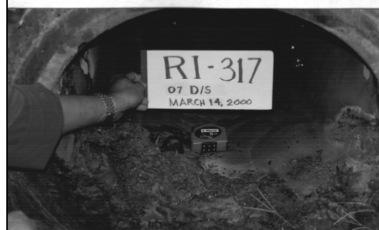
Figure 5. Section of 810 mm line 317, horizontal most section (back of cooling tower).
