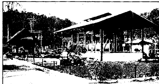
Figure 8. Fang 300 kW Modular OEC Binary Geothermal Power
